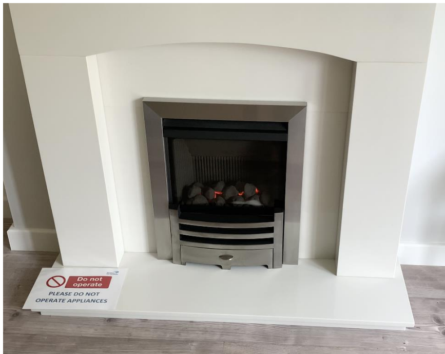
Figure 6, a purpose designed and manufactured 100% hydrogen powered gas fire
