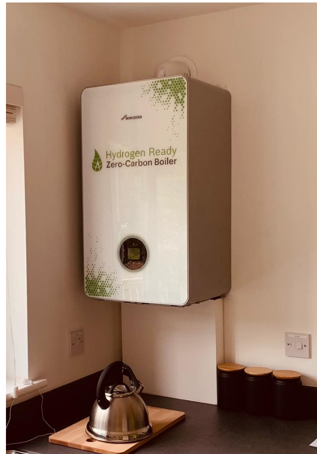
Figure 3, two domestic boilers powered by 100% hydrogen
