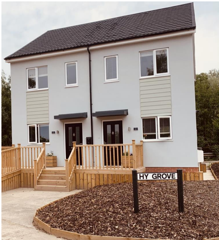
Figure 2, two domestic houses being supplied with 100% hydrogen
