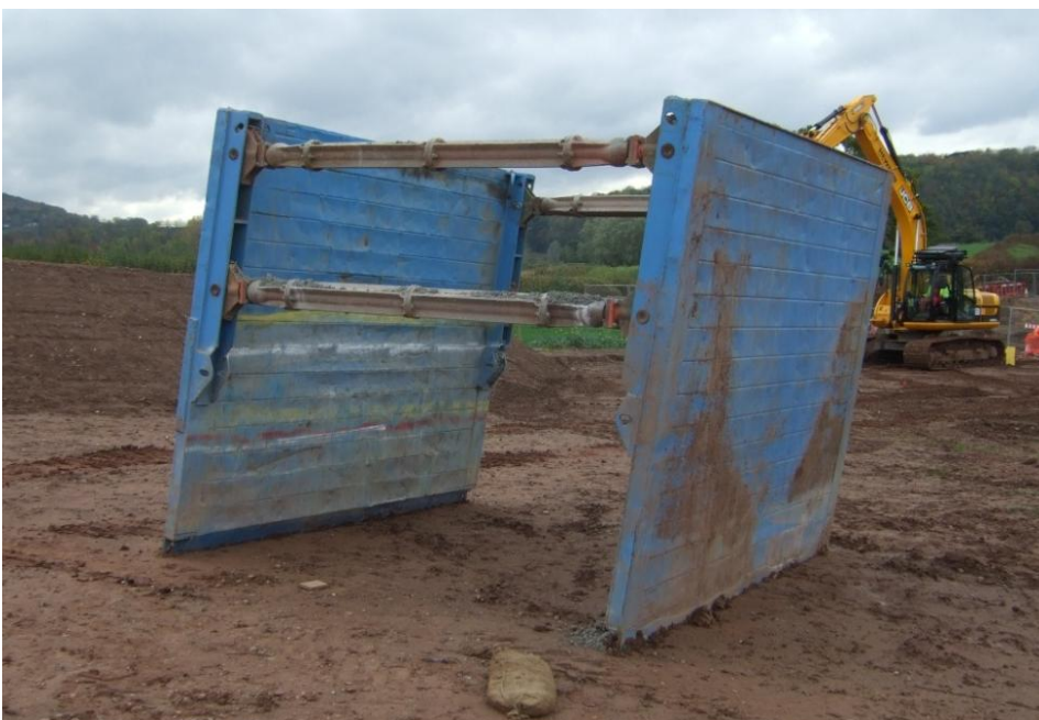
Figure 36 – A section of trench box shoring (out of the trench)
