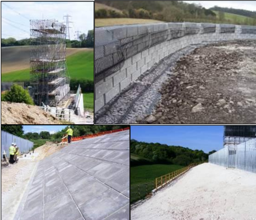
Figure 30 – Retaining walls and earthworks (enabling works)
