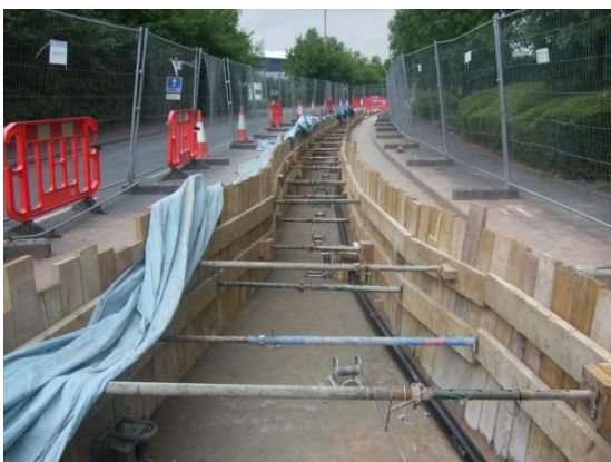
Figure 42 – EHV cable trench in a public road (north-west England)
