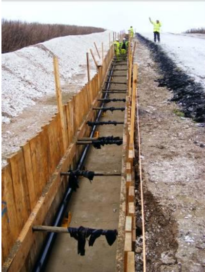
Figure 41 – Cable installation in an open cut trench
