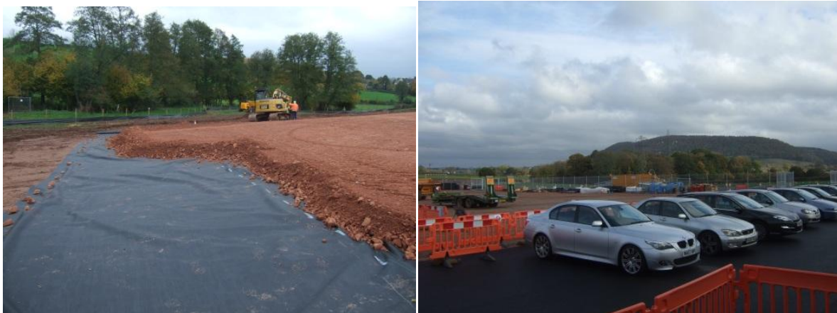
Figure 28 – Site storage/laydown area and site administration
