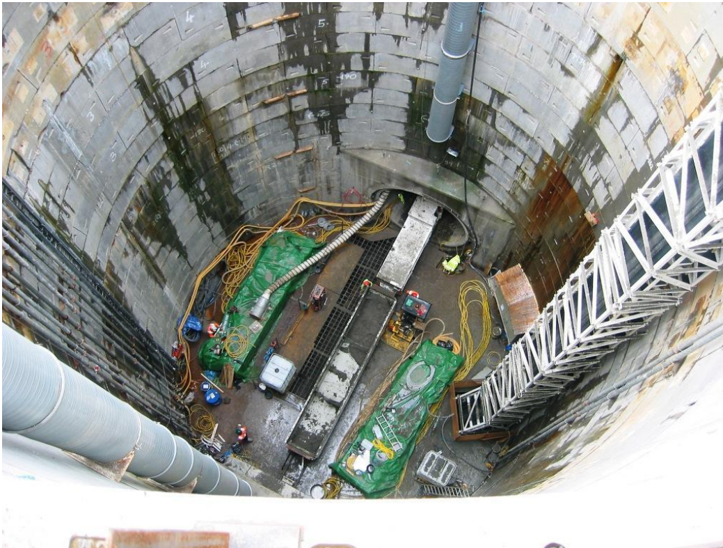
Figure 69 – Central shaft with tunnel constructed in both directions
