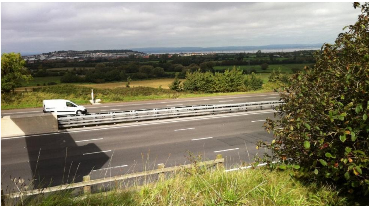
Figure 3 – M5 Motorway looking north towards Portbury
