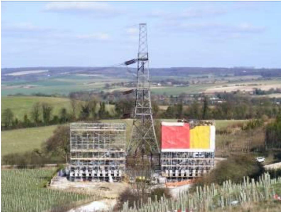
Figure 23 – Weatherproof enclosure for cable termination assembly
