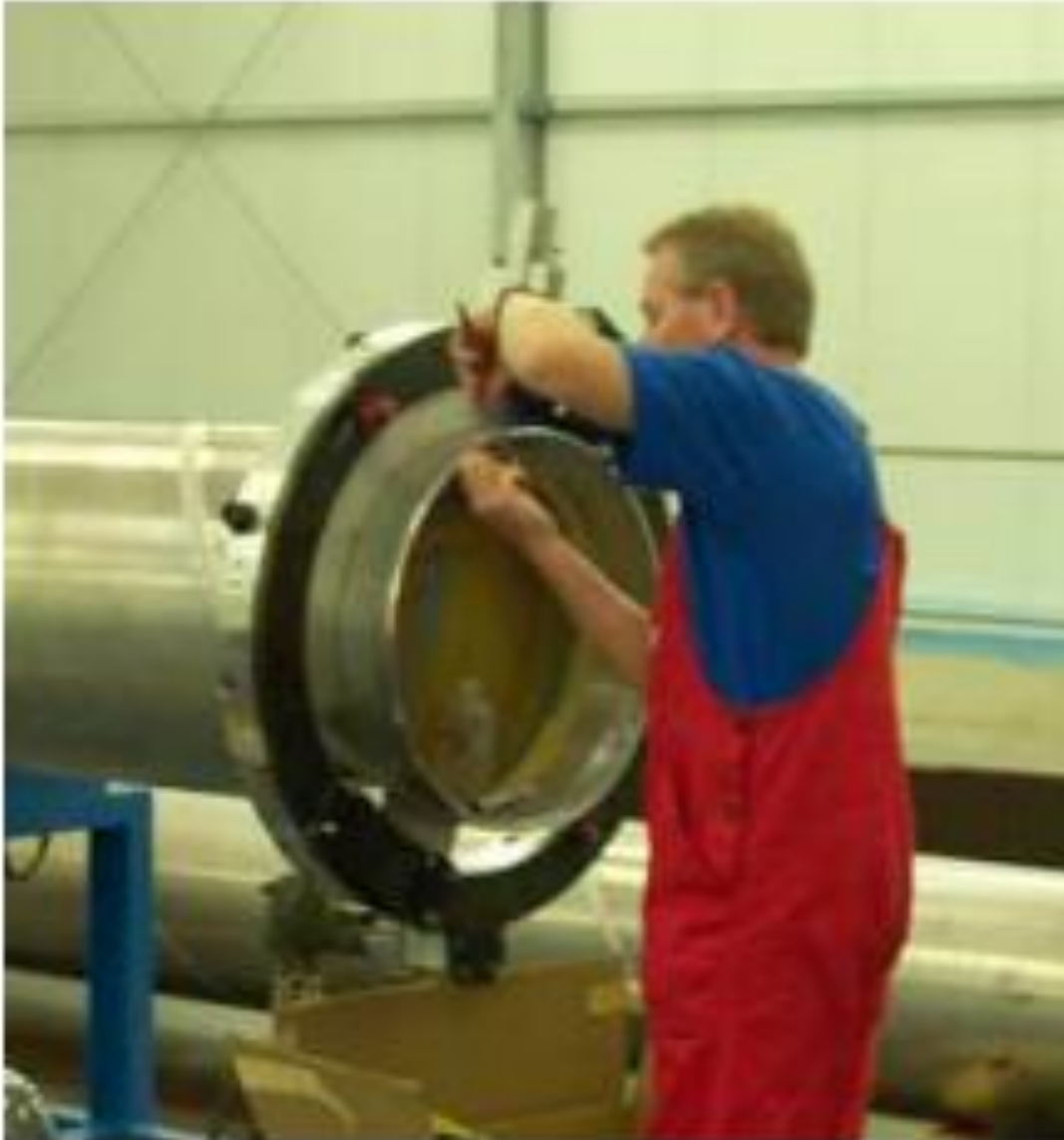
Figure 61 – GIL weld edge preparation prior to connection
