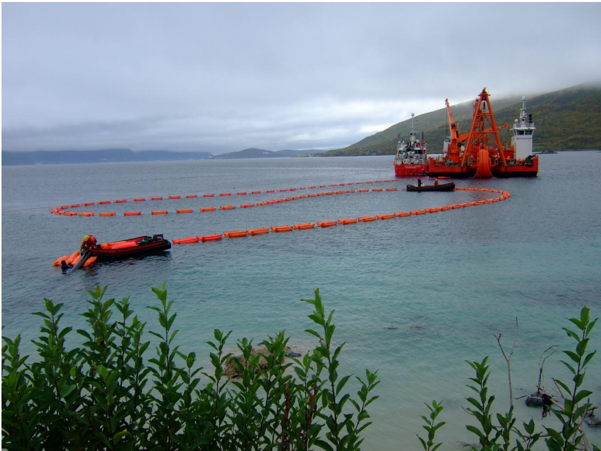
Figure 55 – Cable laying vessel shore landing installation
