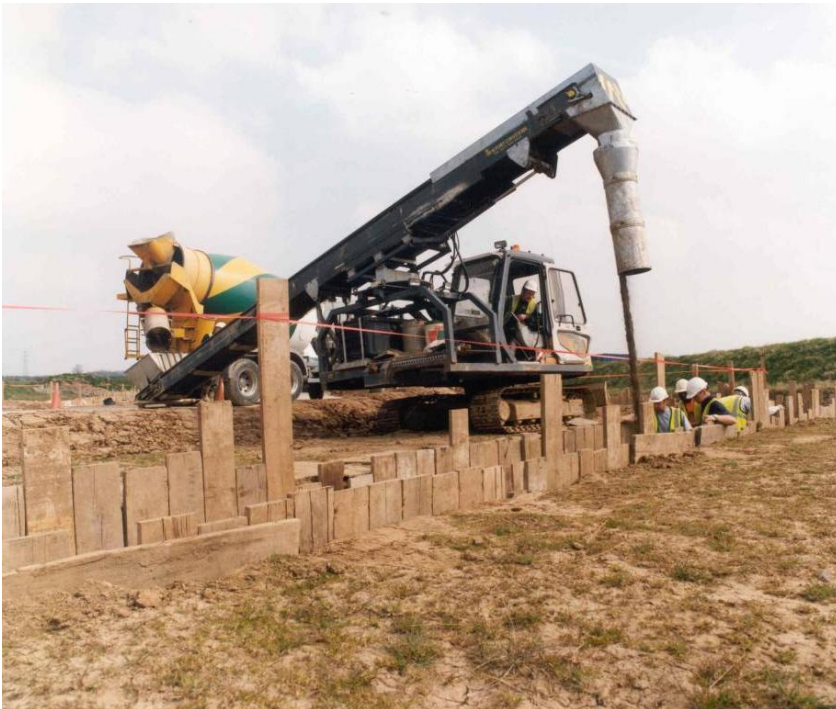
Figure 43 – Delivery of cement bound sand to the cable trench
