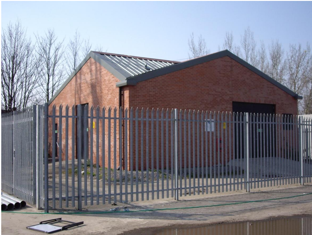
Figure 72 – Completed shaft head-house, within a secure compound
