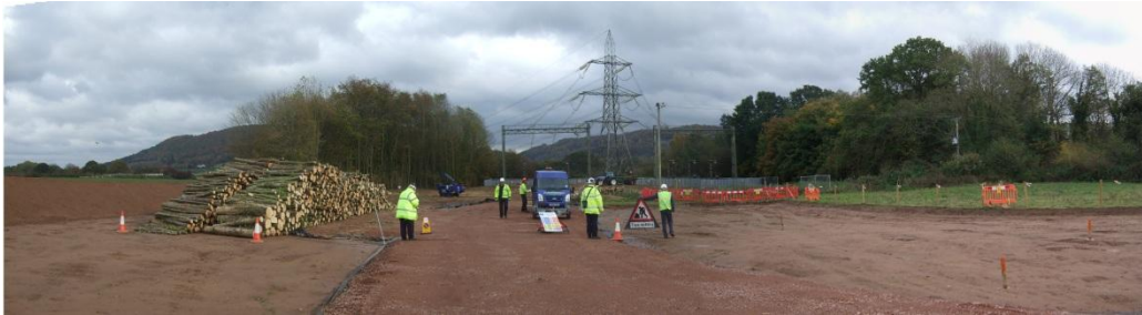
Figure 34 – Clearing woodland from the swathe (Ross-on-Wye 400kV)
