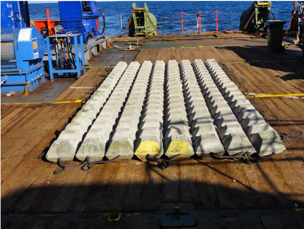
Figure 56 – Concrete mattress (on board ship, prior to deployment)
