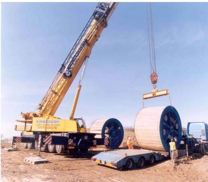
Figure 40 – Offloading cable drums
