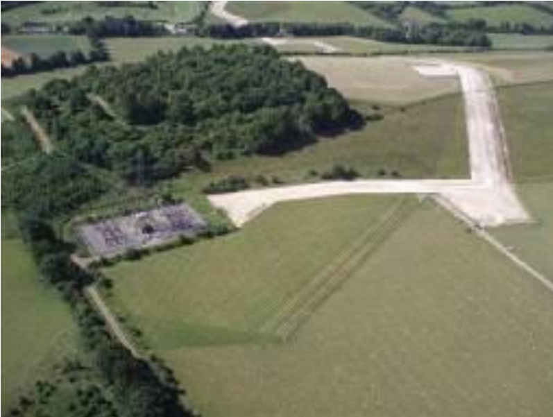
Figure 24 – Moulsoford Down 400kV SEC near Goring
