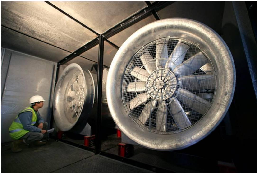
Figure 46 – Air cooling fans during installation
