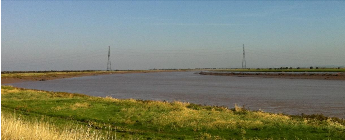
Figure 9 – Combwich Reach river crossing
