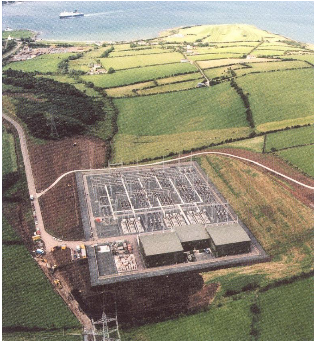
Figure 58 – Ballycronan More 500MW CSC converter station
