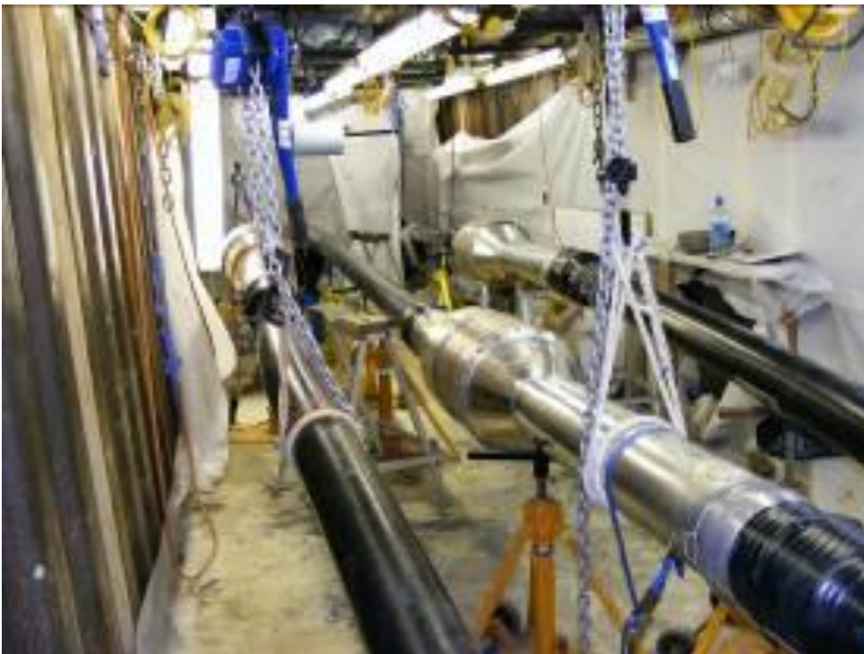
Figure 20 – 400kV cable joints near completion of the jointing process
