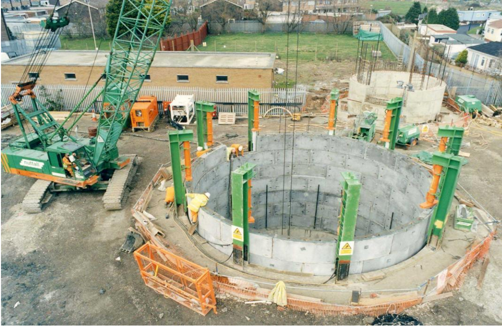
Figure 67 – Hydraulic jacks on caisson technique shaft construction
