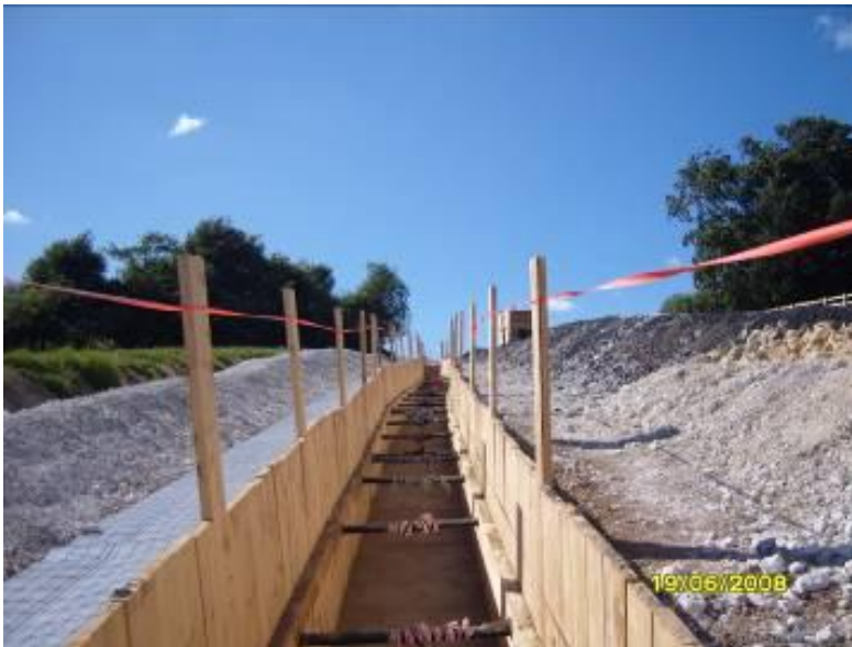
Figure 37 – A close-timbered cable trench
