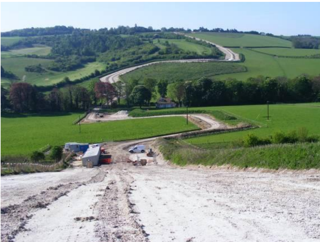
Figure 35 – 400kV cable swathe at the Goring Gap
