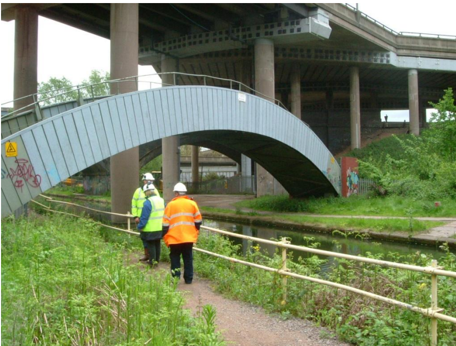
Figure 29 – Steel cable bridge over a Birmingham canal (special construction)
