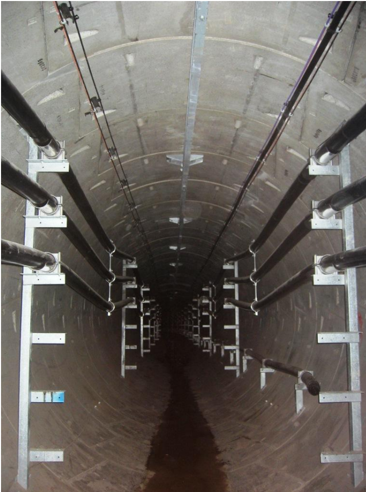
Figure 71 – Completed tunnel: vehicle monorail and power cables installed
