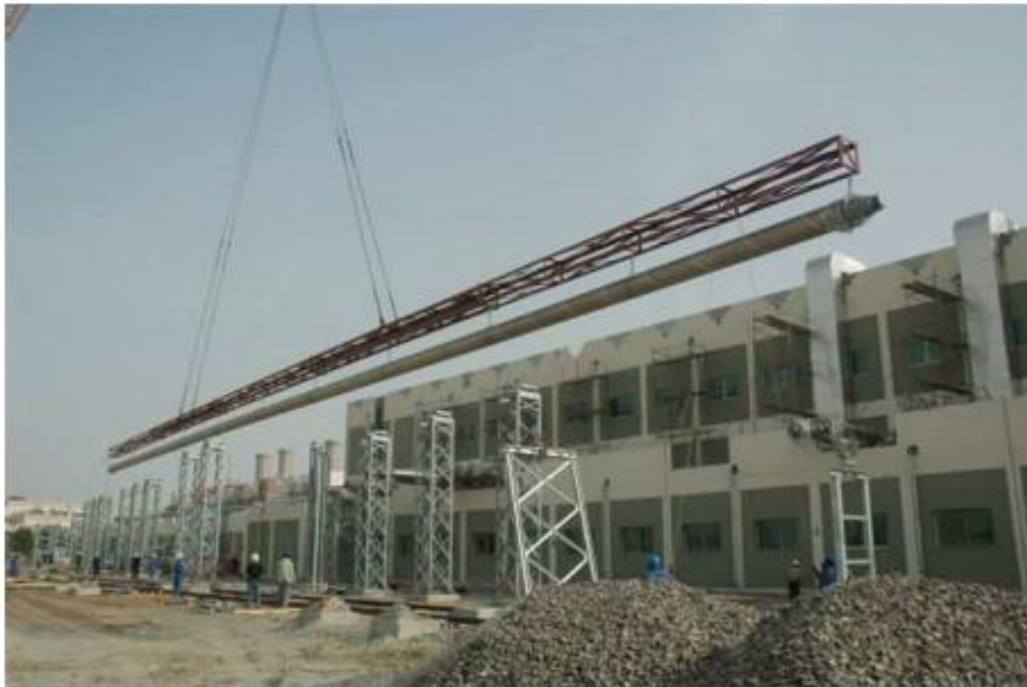
Figure 62 – GIL segment being lifted into position
