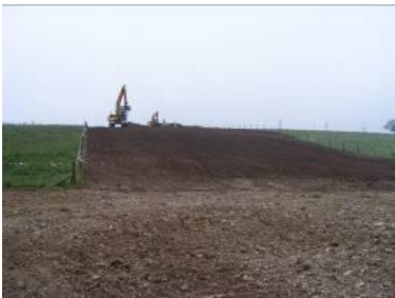
Figure 44 – Topsoil replacement
