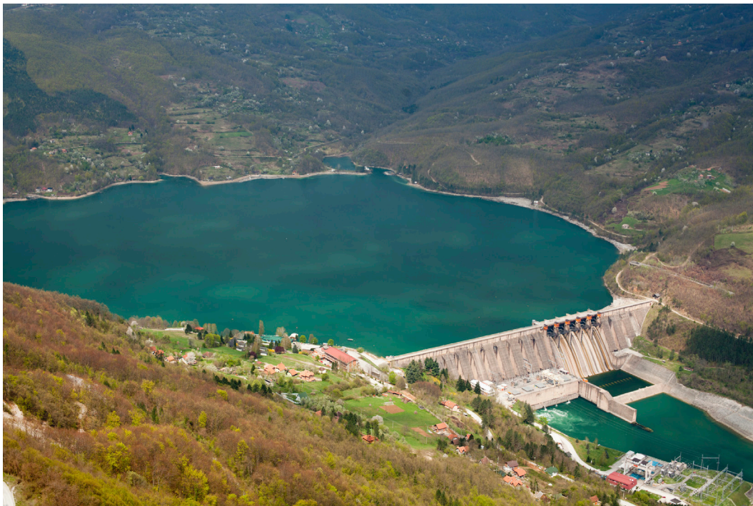
River Drina hydroelectric power station, border of Serbia and Bosnia
