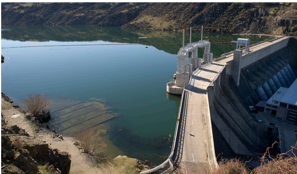
Roxburgh hydroelectric power station, New Zealand
