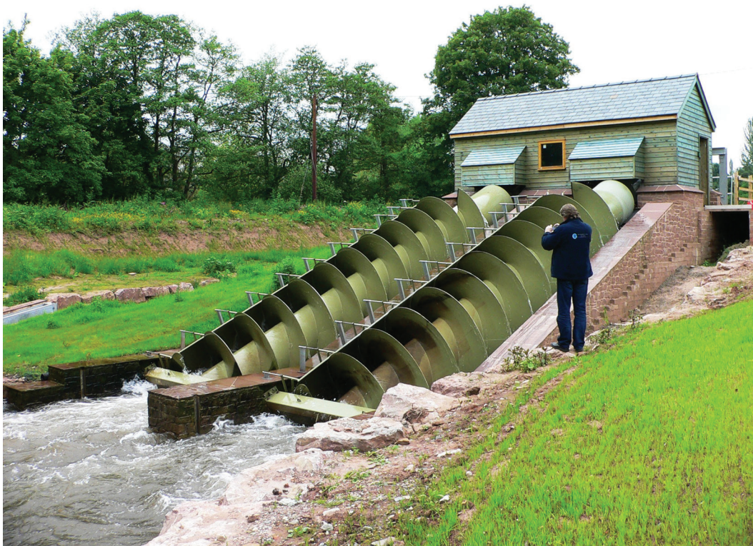
Archimedean screw turbine, Osbaston, Wales (with kind permission of MannPower Consulting Ltd)
